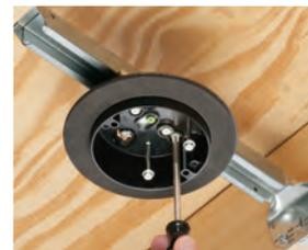
**4** Tighten box screw to lock box in position.
