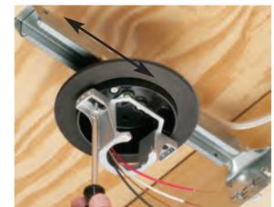
**5** Remove captive installation screws to install fan/fixture mounting bracket (drywall installation not shown).
