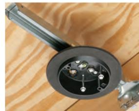
**3** Loosen box screw (provided). Slide box along bracket to position box between joists.
