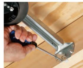
**2** Remove 'parked' screws from both sides of bracket. Use to attach bracket to joists.
