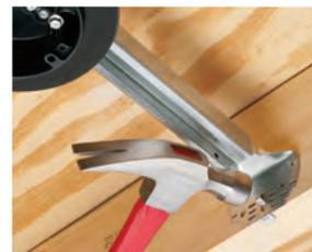
**1** Nail 'tooth' to joist to hold bracket in place temporarily.
